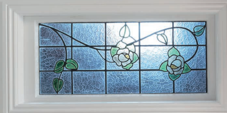
PHOTO: Reclaimed stained glass reused as loft hatch to bring natural light from roof light. Absolute Project Management. Photo credit- Moon Street Studio
